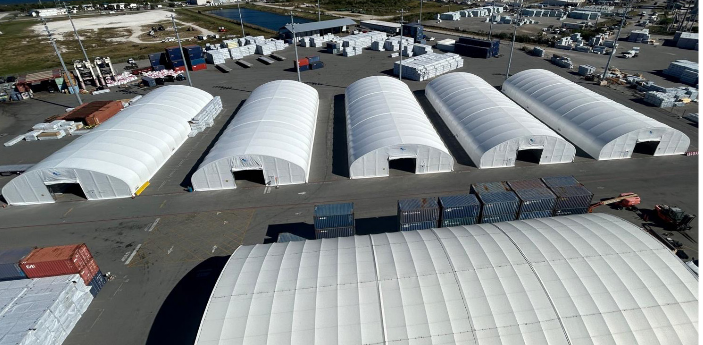
Aerial shot of the new warehouses built at Canaveral Cargo Terminal
